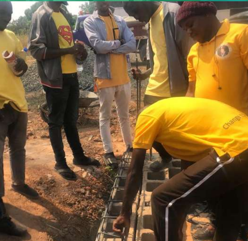
MASONRY FIELD WORK
