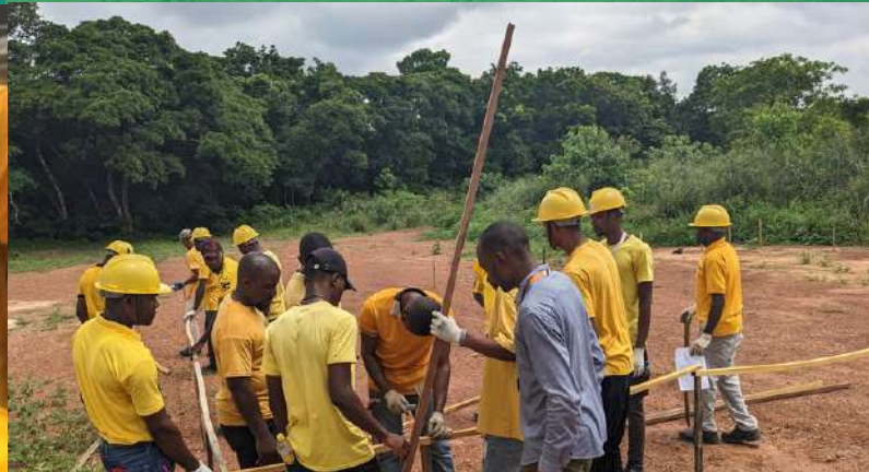
MASONRY FIELD WORK
